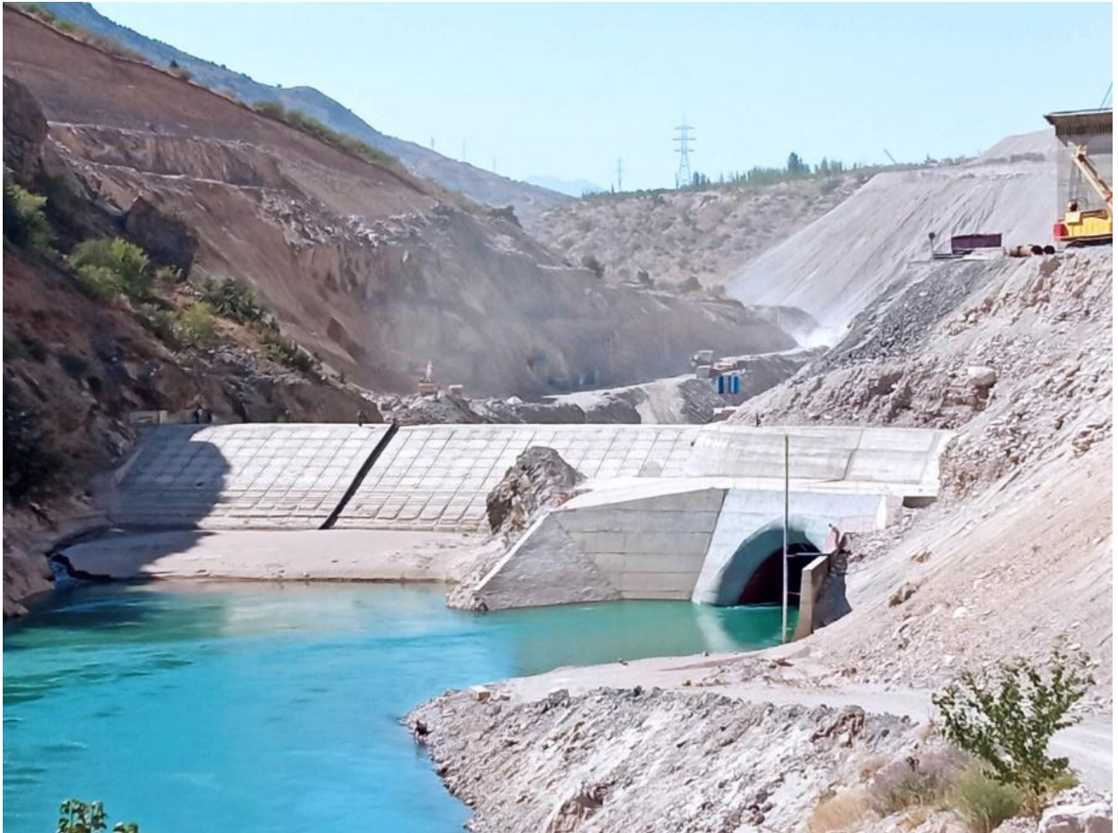
Figure 12. Construction Site of the Lower Chatkal Hydropower Plant, Uzbekistan. Source: Rivers without Boundaries.
