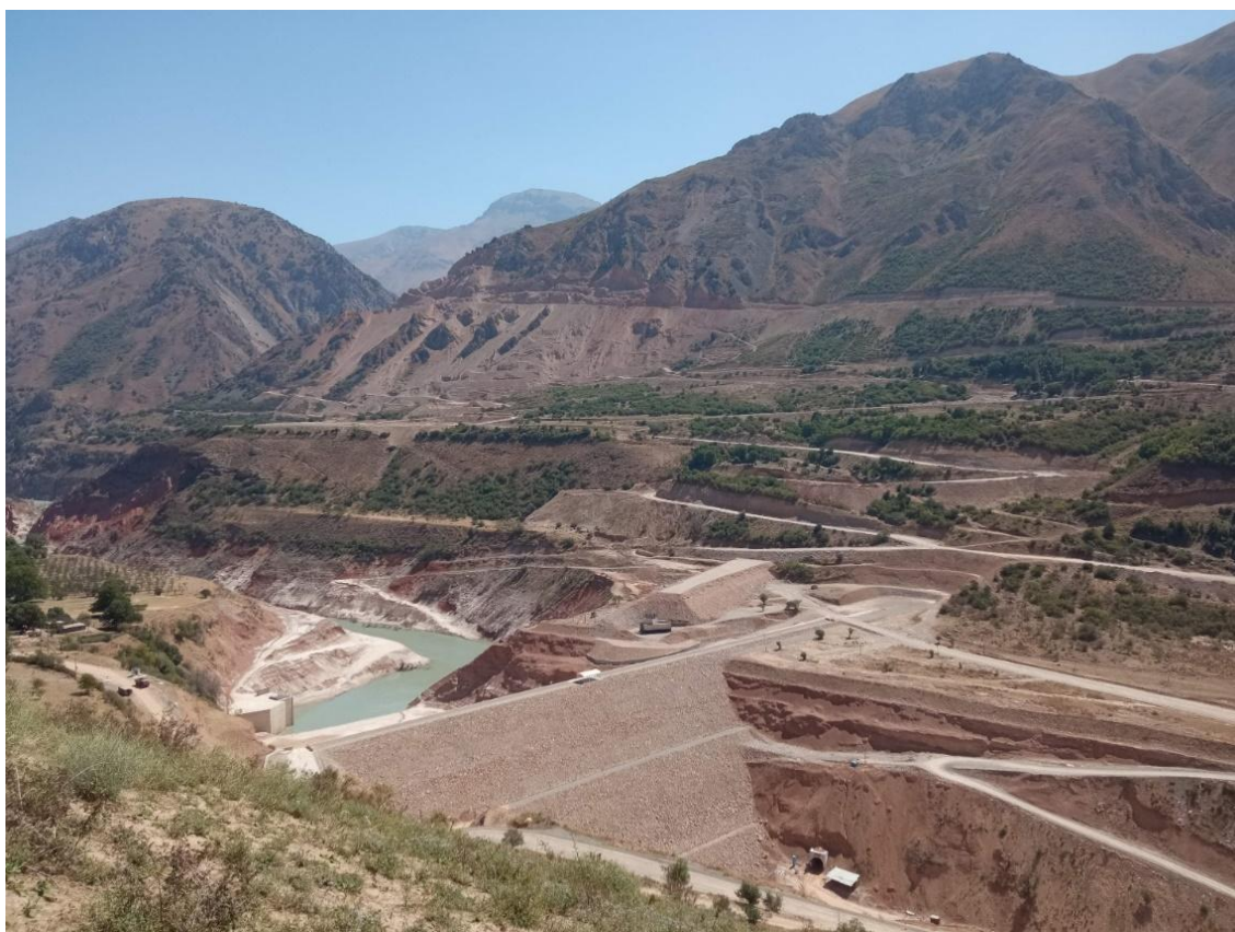
Figure 14. Pskem HPP Construction in the Pskem River Valley, 2023. Source: Rivers without Boundaries .
