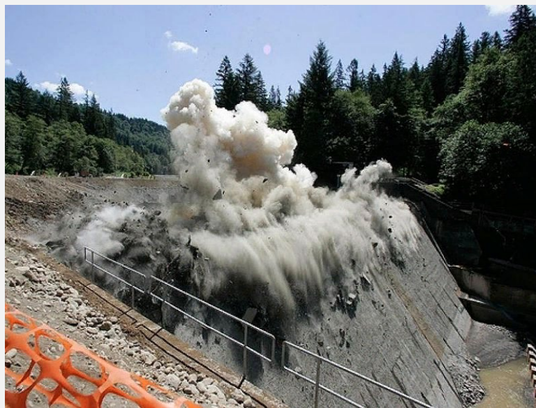
The Marmot Dam on the Sandy River in Oregon was demolished in 2007 using dynamite
